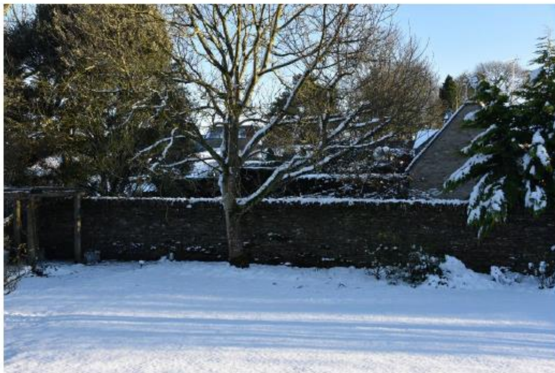
RECENT PHOTO CURRENT EXTENSION (NW ELEVATION)
